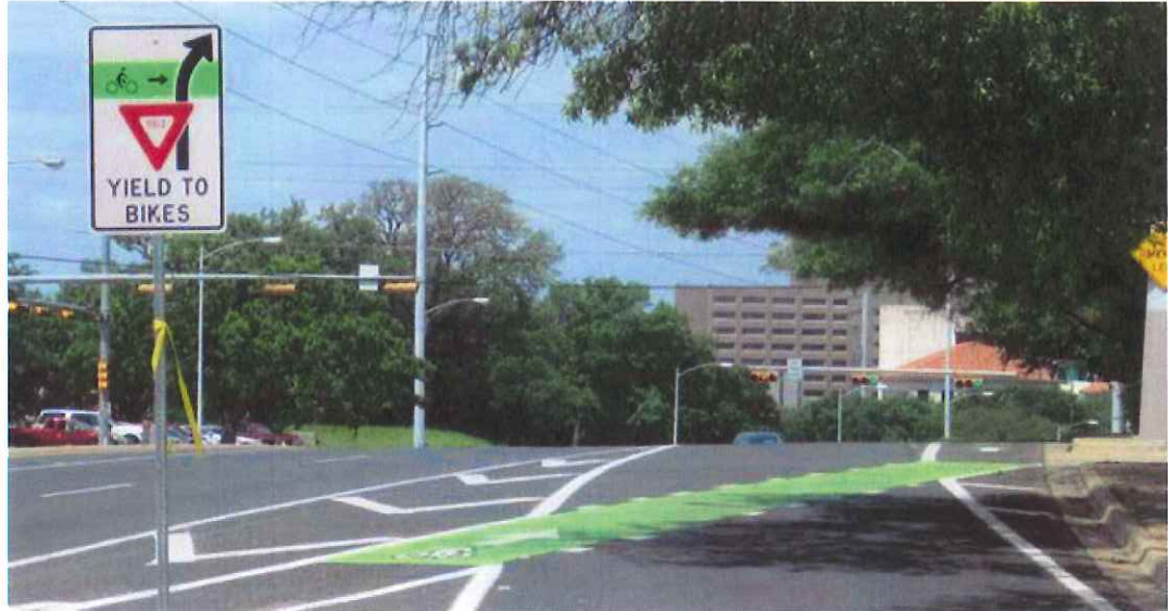
Figure 17: Example of Colored bicycle lanes and Signage in Conflict Areas 12
