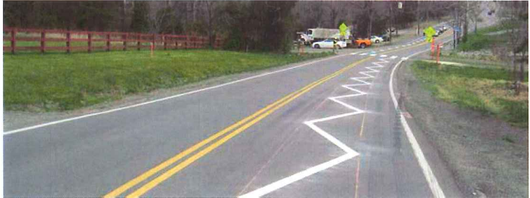
Figure 15: Example of Zigzag Striping to Alert Motorists to Reduce Speed 10
